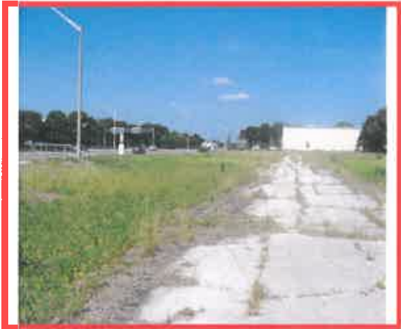
Photo of Parcel Facing West
